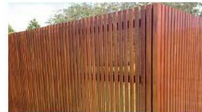
6. Timber slatted external plant enclosure
