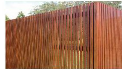
6. Timber slatted external plant enclosure
